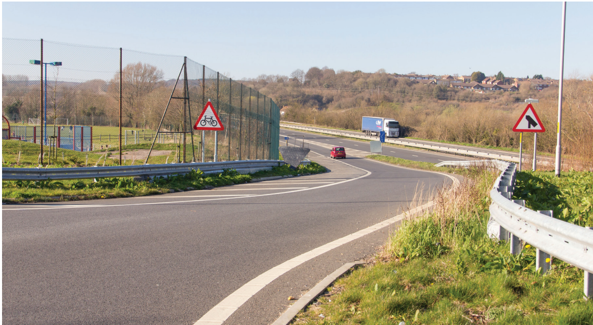
Figure 1.2 A2 London Bound On-Slip Road
